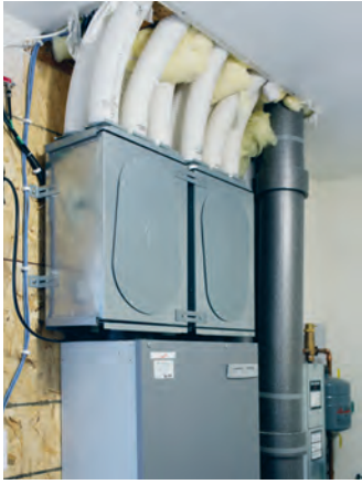
An installed Zehnder CleanAir 350 ventilation system
