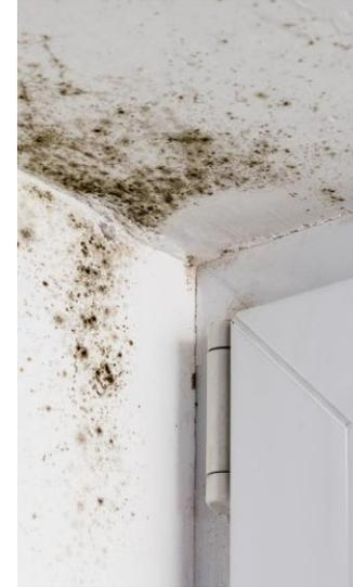
A building with an airtight building envelope without ventilation is not functioning – mould is attacking the building fabric
