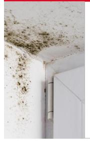
A building with an airtight building envelope without ventilation is not functioning – mould is attacking the building fabric
